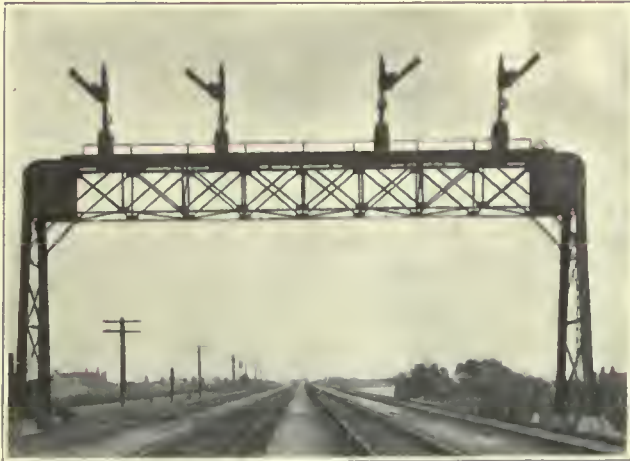
FIG. 284. SIGNALS. Standard signal bridge on the Pittsburgh, Fort Wayne & Chicago Railway, near Drexel Avenue.
